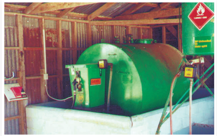
The most effective bunds are able to contain large volume spills, and are under cover to prevent them filling with rainwater
