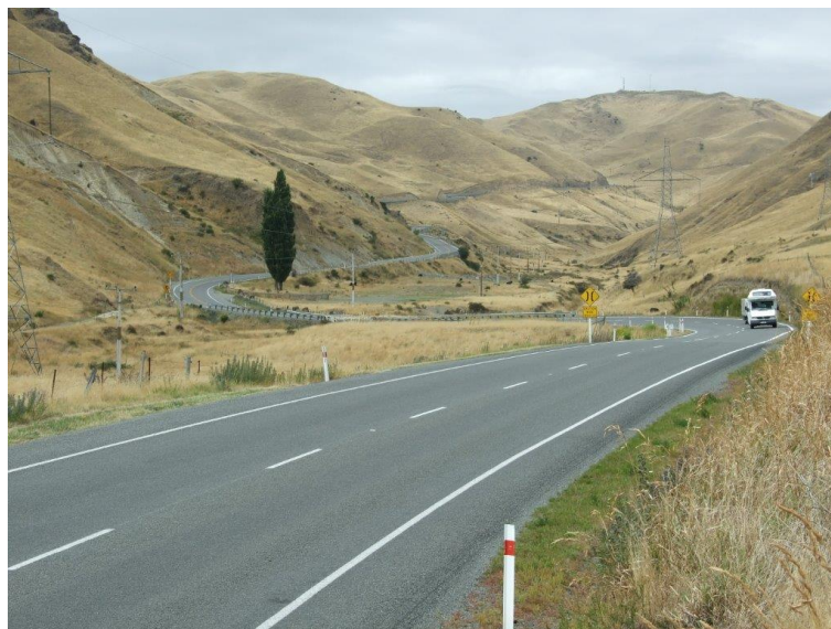
Puka Puka Weld Pass SH1, Marlborough
