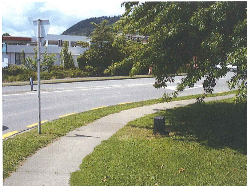
Photograph 1 : Looking west on Boundary Road showing vegetation obscuring signage
