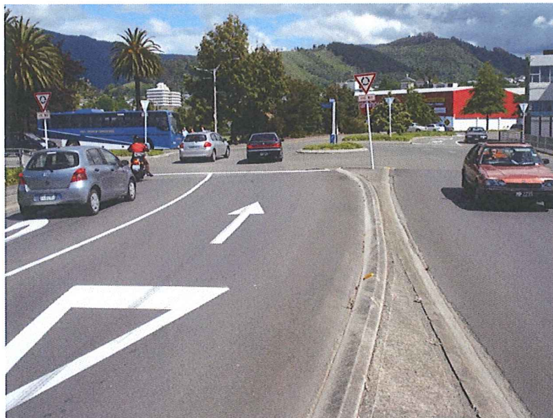
Photograph 6 : Looking south on Haven Road showing poor deflection for through traffic on this approach
