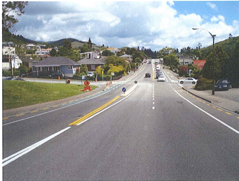
Photograph 3 : Looking south on Waimea Road showing vehicle waiting to turn right from Motueka Street and one vehicle having just completed movement
