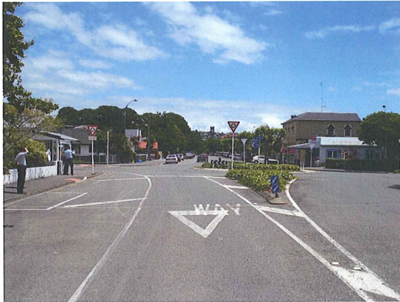
Photograph 8 : Looking west on Nile Street showing poor deflection for through traffic. The photo also shows the lack of islands on the left side of the lane that would assist in channelizing the traffic. This is typical of the whole intersection
