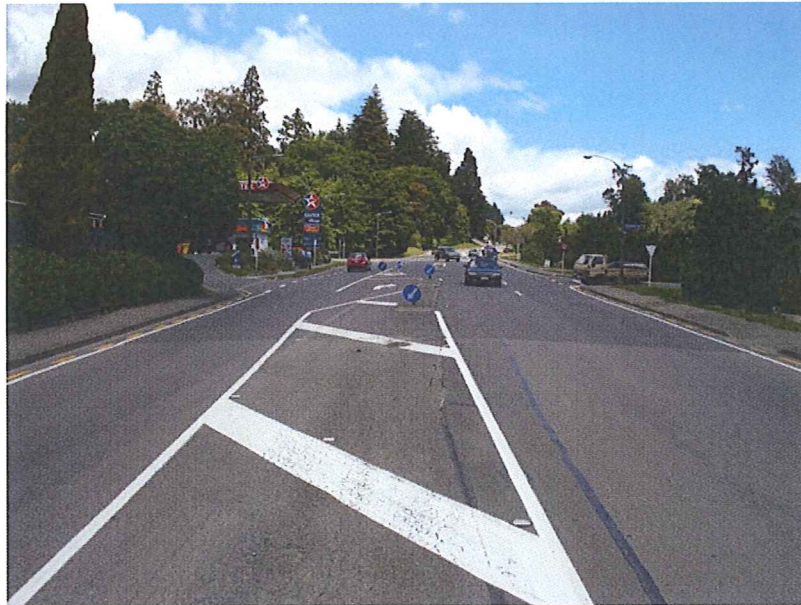
Photograph 2 : Looking south showing complexity of intersection layout with poorly delineated islands
