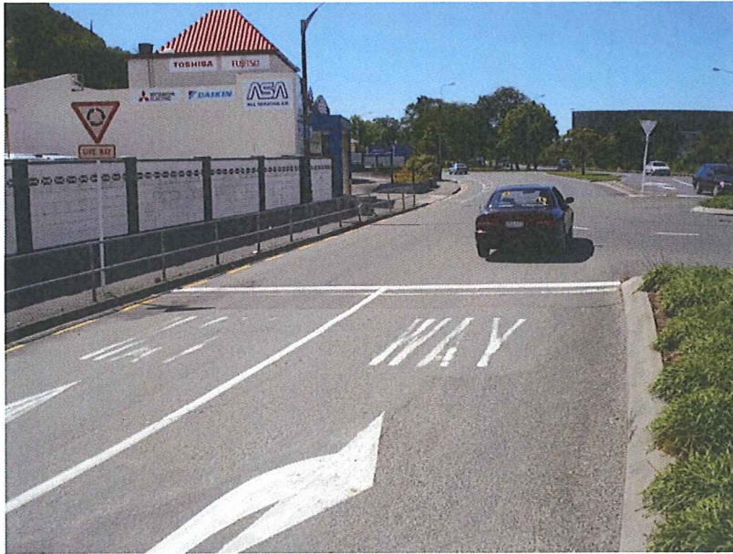
Photograph 5 : Looking north on Haven Road showing poor deflection for through traffic on this approach
