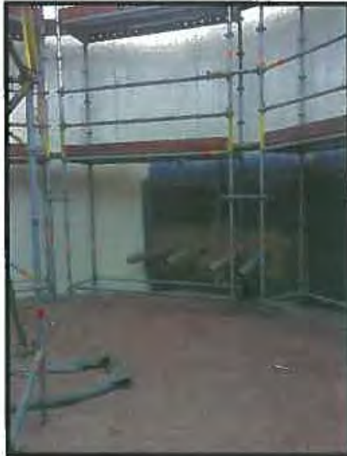
Figure 3: Tank A Coating partially applied
