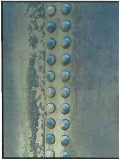
Figure 2: Riveted joint after preparation
