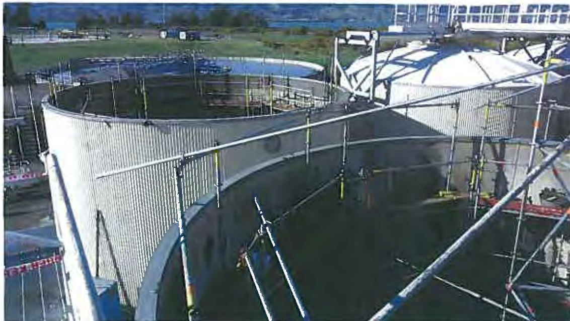
Figure 1: A-Train Sludge tanks with ring fitted
