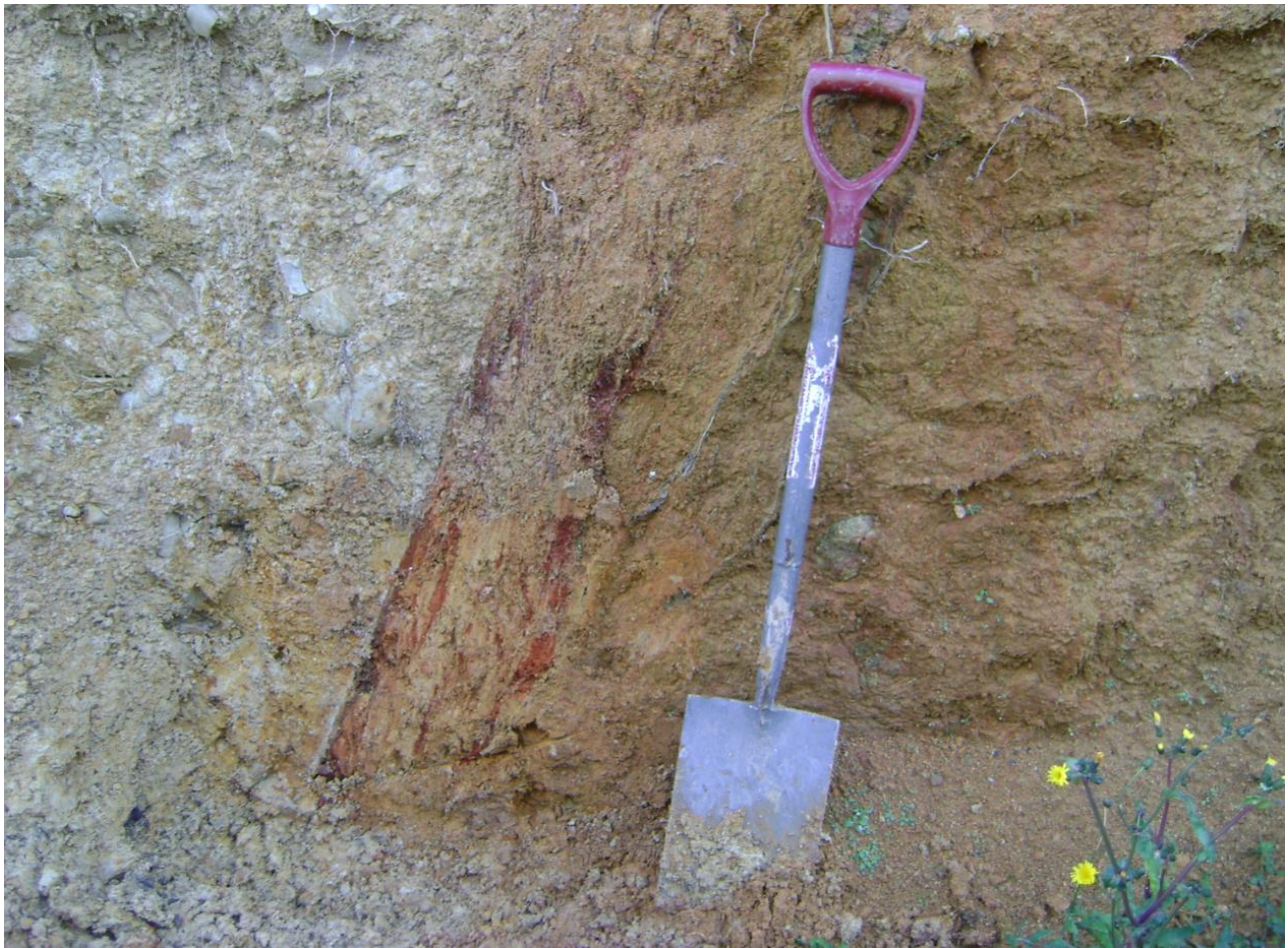
Figure 8.16 Nasty surprise: Picture shows evidence of major fault rupture through an area that is currently identified for the extension of York Valley.
