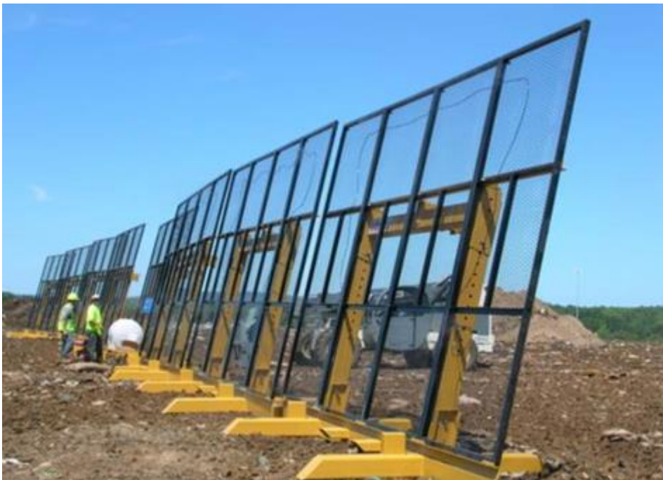
Figure 9.6.1 Debris catch fences to improve mitigation of wind-blown debris
