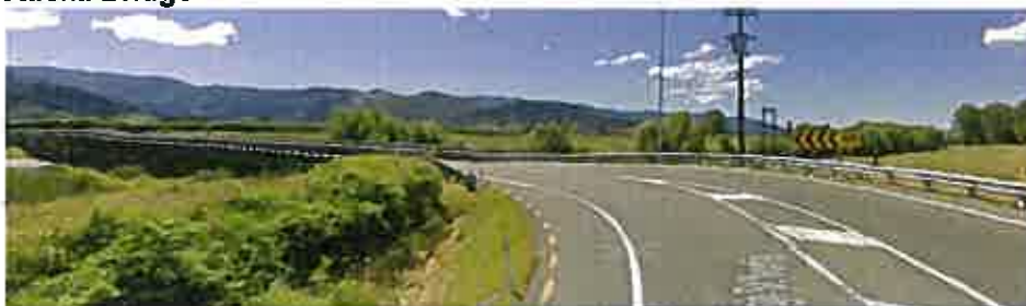
SH60 Motueka Bridge approaching from Motueka
