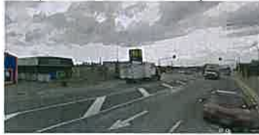
SH6 – Gladstone Road/Queen Street intersection (looking north)
