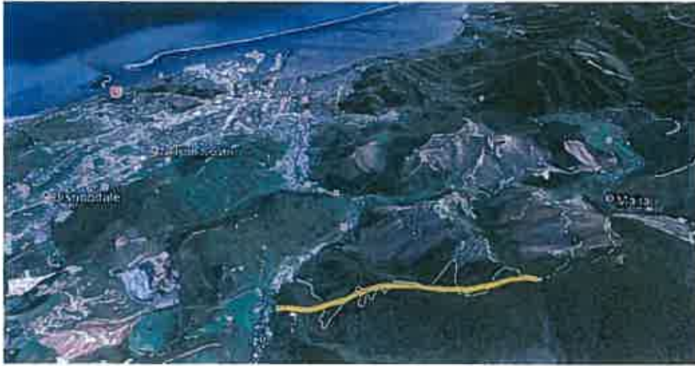
View north overlooking gondola site
