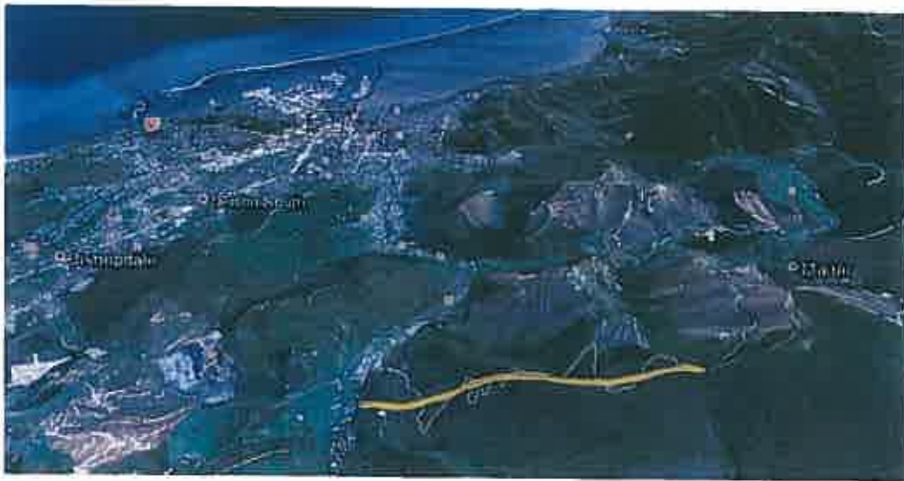
View north overlooking gondola site
