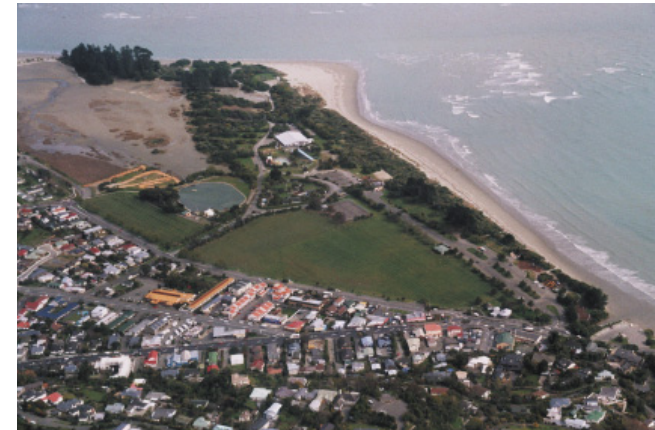
Aerial oblique of Tahunanui Beach and the Back Beach Embayment. The relatively unmodified natural character of this area is of increasing significance as urban growth in Nelson South and Richmond is placing it at the centre of the wider urban area.
