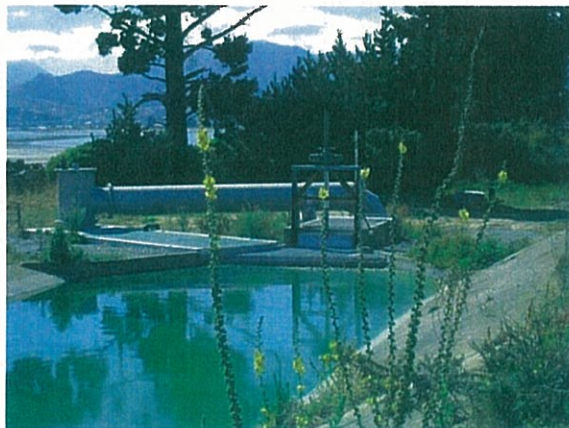
Figure 3 The installation of the booster pump on the outfall pipeline doubles the peak capacity of the outfall
