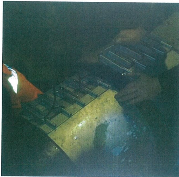
Figure 1 Remedial work to gibault damaged during location
