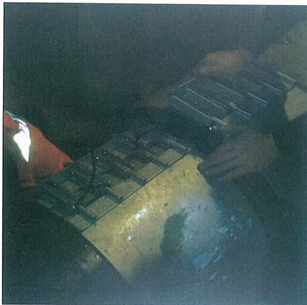
Figure 1 Remedial work to gibault damaged during location
