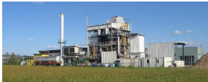
Figure Z - Güssing 2MWe gasification and CHP plant
