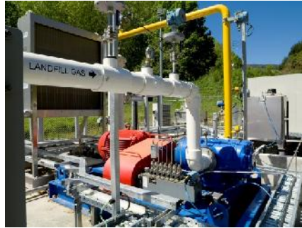
Figure Y - Nelson Hospital Landfill Gas Plant
