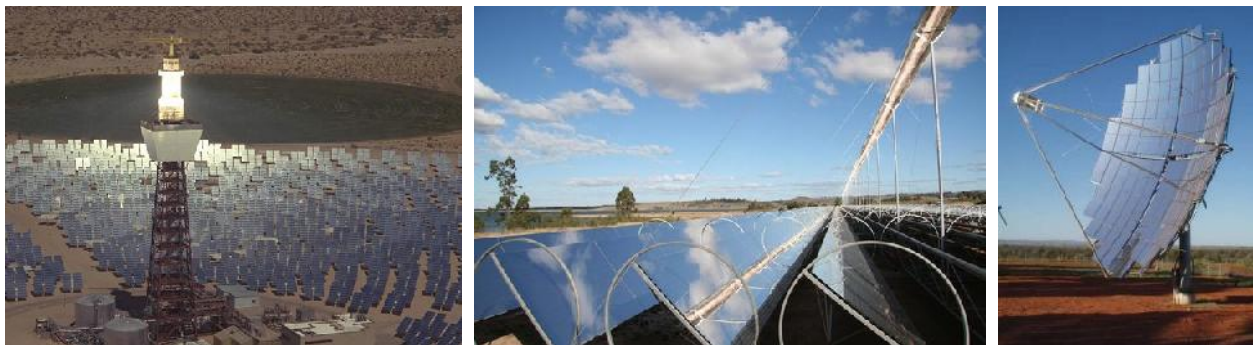
Figure O - CSP Technologies – Power Tower with Heliostat Mirrors 14 , Linear Fresnel Reflector 15 , Concentrated PV 16
