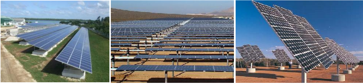
Figure M - Examples of Solar Farm Mounting Systems – Fixed (Concrete Slab) 11 , Single Axis Tracker 12 and Dual Axis Tracker 13
