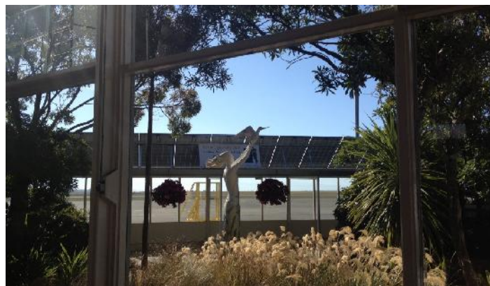
Figure D - 11 kW Solar PV Array at Nelson Airport
