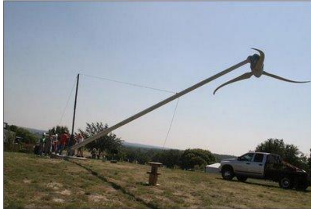
Figure H – 1.8kW Skystream Wind Turbine Being Installed
