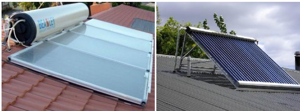
Figure J - Example of Flat Panel and Evacuated Tube SHW Systems
