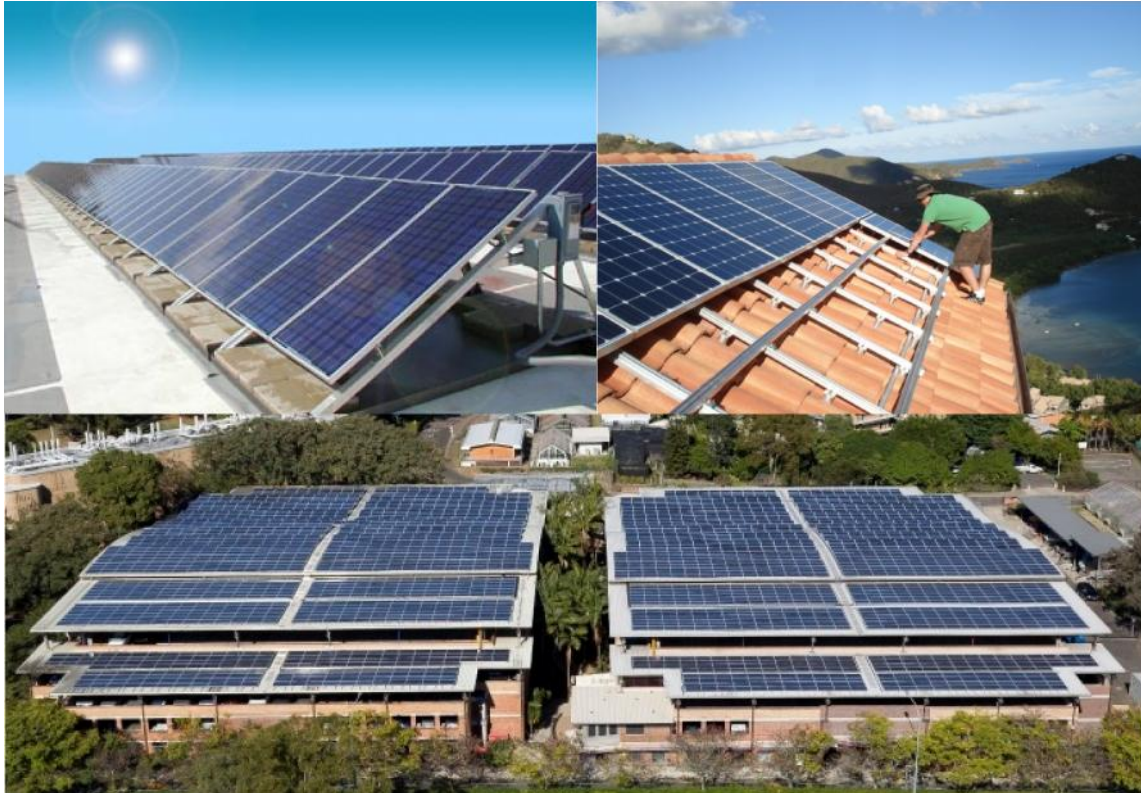
Figure L - Rooftop PV System Examples - Commercial, Residential and University of Queensland 1.2MW 10
