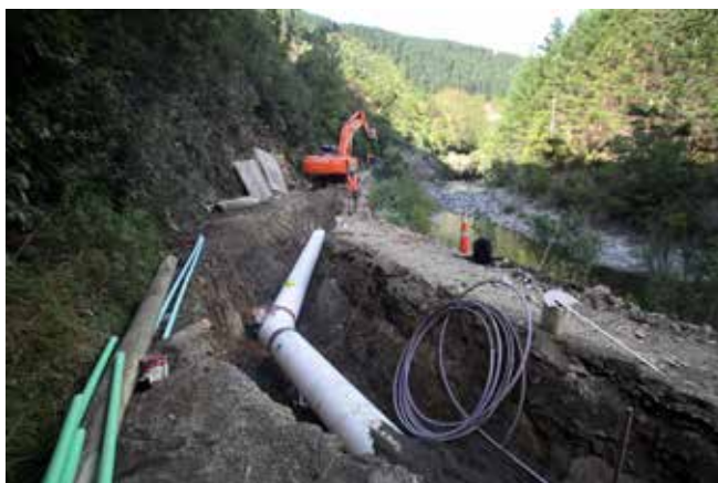
Construction of the duplicate pipeline from the Maitai dam to the water treatment plant
