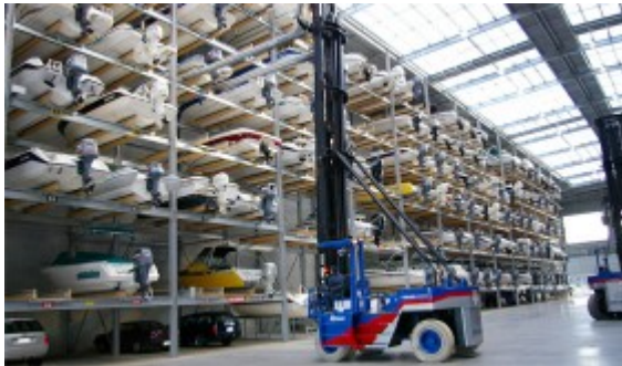
Figure 2 Example of a Large Scale Dry Stack
