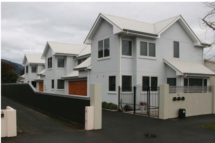
Figure A. The roof forms and fencing in this townhouse complex pick up on the local suburban details.
