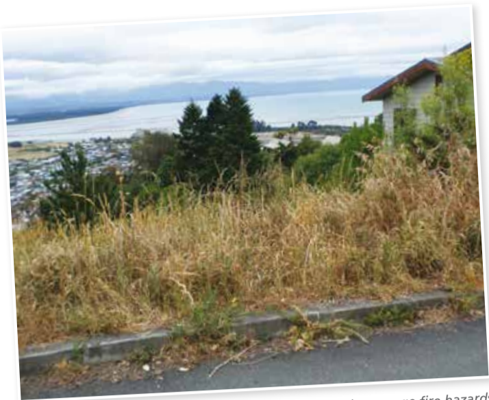
Dry overgrowth and scrubs need to be cut back to help manage fire hazards
