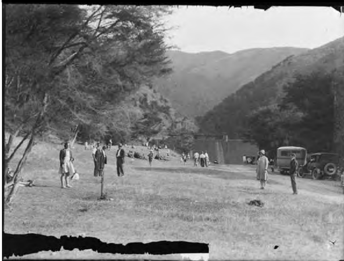
Figure 10: The Brook Street Reservoir in about the 1920s
