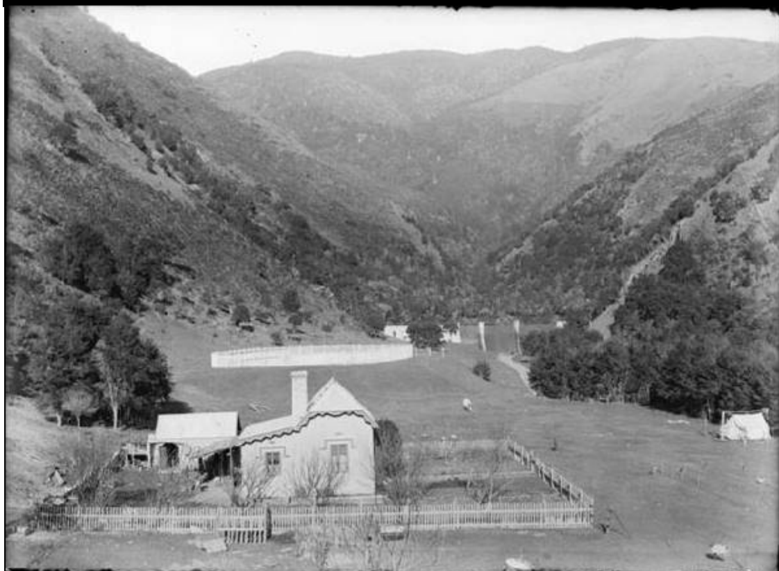
Figure 8: Brook Street Reservoir and Cottage 1902-1908
