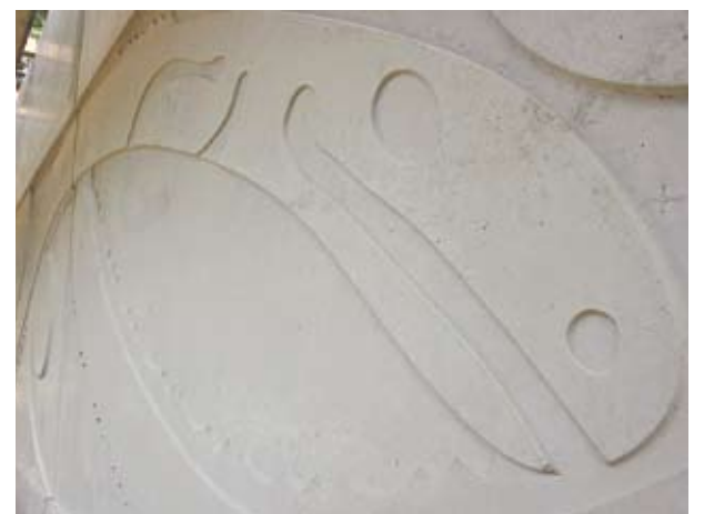
Nelson carver Brian Flintoff designed the eel motif for the Normanby Bridge walkway.
