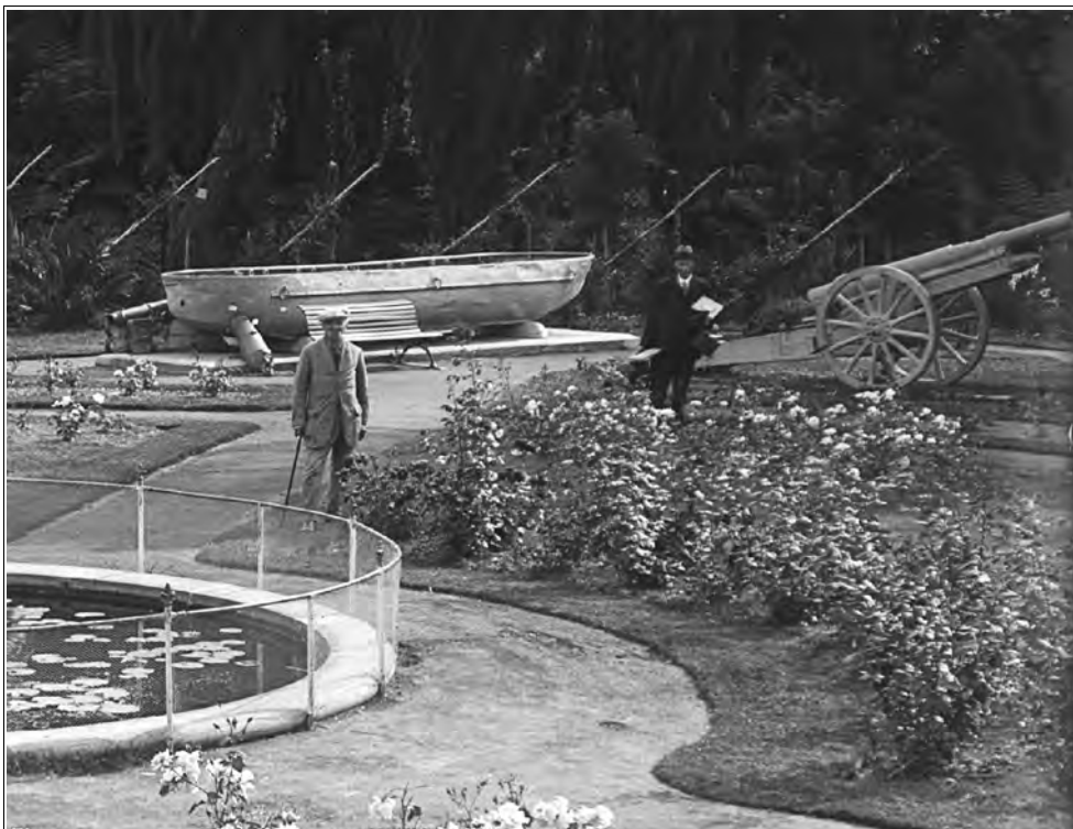
Figure 2.22 Exploded detail showing the Turkish Pontoon with a Field Gun on right and cannon on the left. These were displayed on the former site of the aviary. Photograph undated but between 1923 and mid 1930s.
