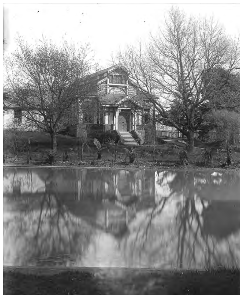
Figure 2.27 View of recently planted pond margins. Ferns and flax visible under Oaks Source: FGG, 333, NPM
