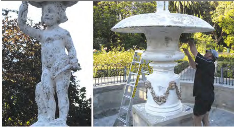
Figure 2.30. Condition of fountain prior to 2010 painting Source: Resene newsletter, 2/2010
