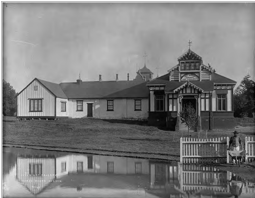
Figure 2.19 Newly completed Bishop Suter Art Gallery and Queen's Gardens Caretaker Mr Edward Christian who was responsible for opening and closing the Gallery and maintaining the grounds c.1899 Source: T182159, NPM
