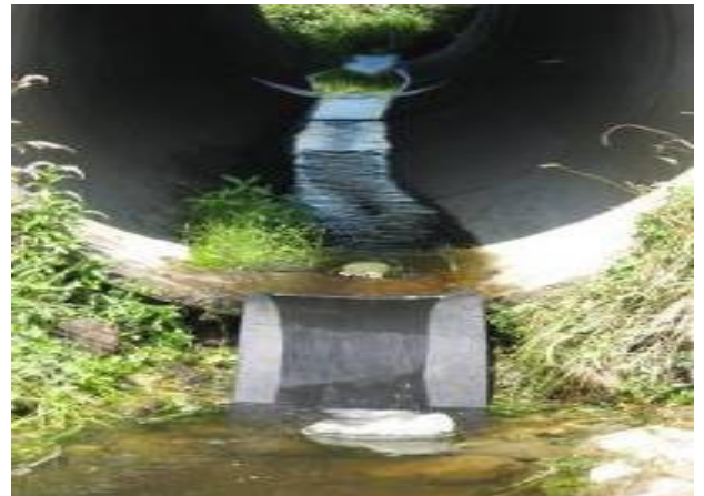
Fig 7 . There are many options for enhancing fish passage including the use of conveyor belt material (Courtesy Trevor James TDC)
