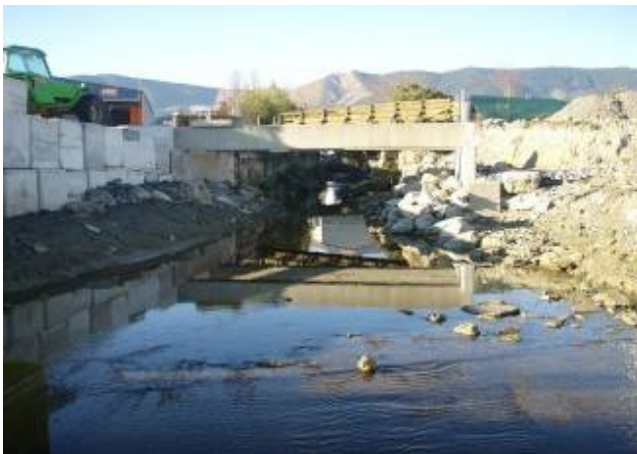
Fig 6 .Saxton Creek immediately upstream from Whakatu Drive enhancement opportunities
