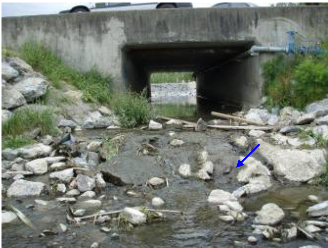
Fig.10 ongoing erosion at the downstream end of the apron could constrain fish passage ( photo taken in 2007)
