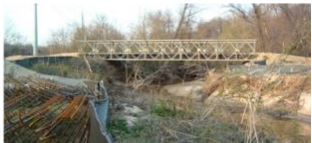
Figure 11-4 Temporary Bridge Crossing
