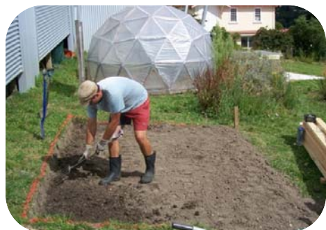
Aaryn Barlow, Master Builder, dug the foundations.
