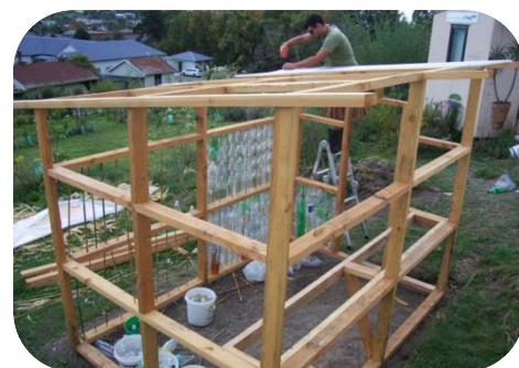
Aaryn put the roof on.
