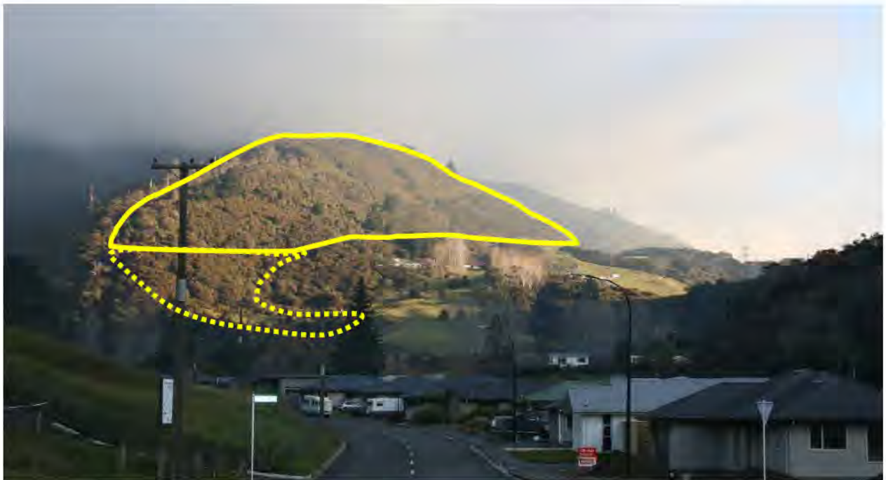
PHOTO 3: Showing ridgeline currently in landscape overlay from Brook Street and approximate location of landscape overlay area. Area that is not visible from major transportation routes or the coast dotted red.
