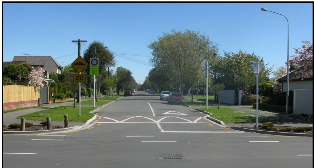
Figure 4-P Intersection Threshold Treatment
