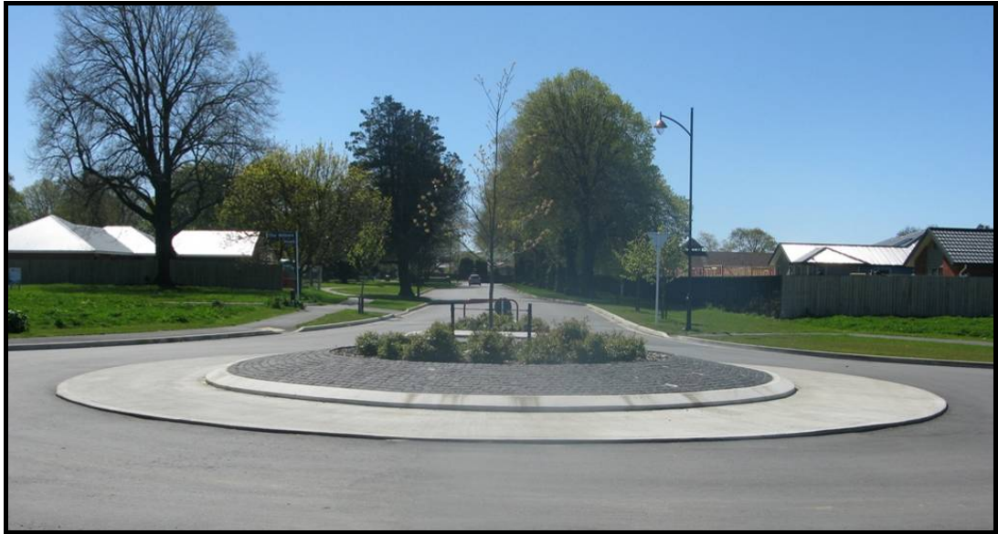
Figure 4-R Roundabout with Semi-Mountable Apron
