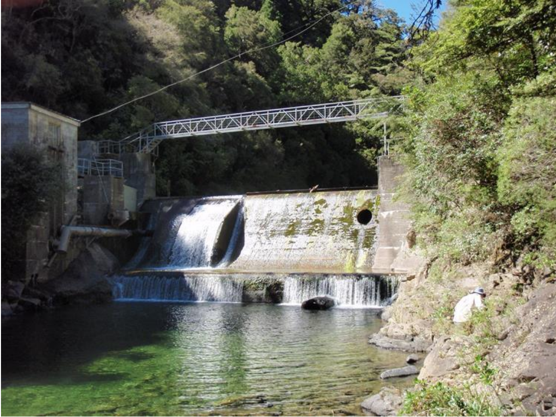
Photo 1. Nelson/Richmond water supply weir, Roding River, Nelson
