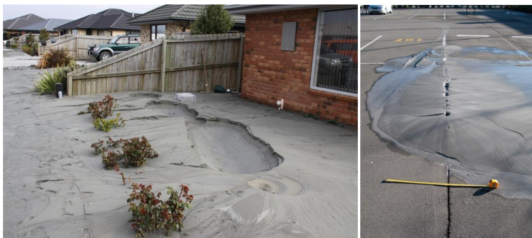
Figure 8 Surface ejection of soil and water as sand boils
