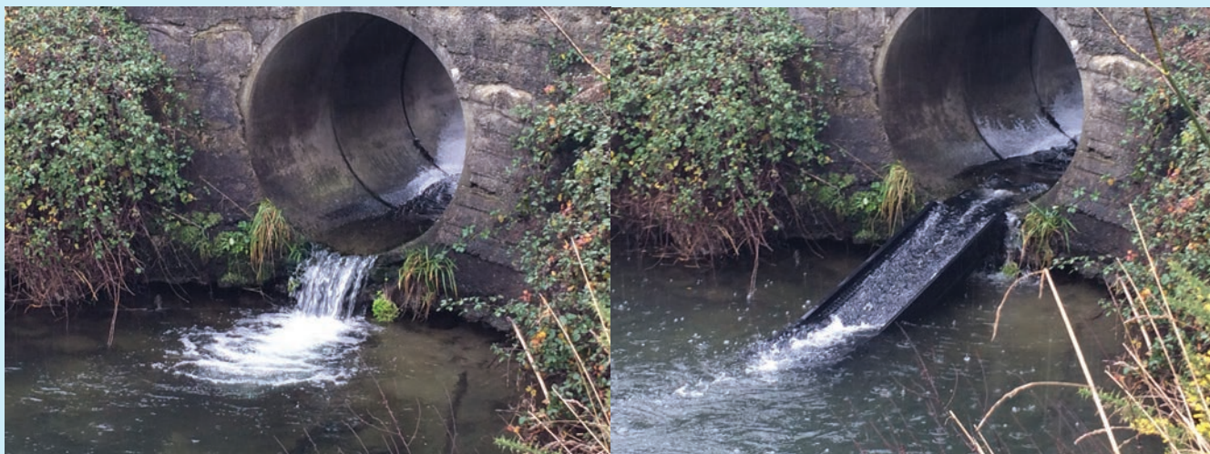
Before and after installation of a fish passage ramp on a perched culvert, Elizabeth Stream.
