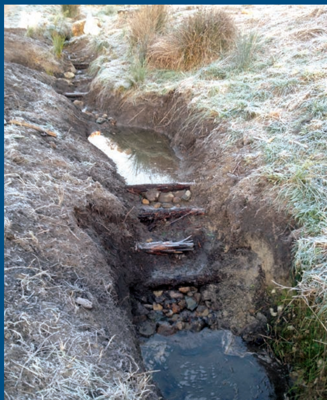
Stream restoration in progress to create fish pool habitat and fish ladders and introduce woody-debris to the stream channel.
