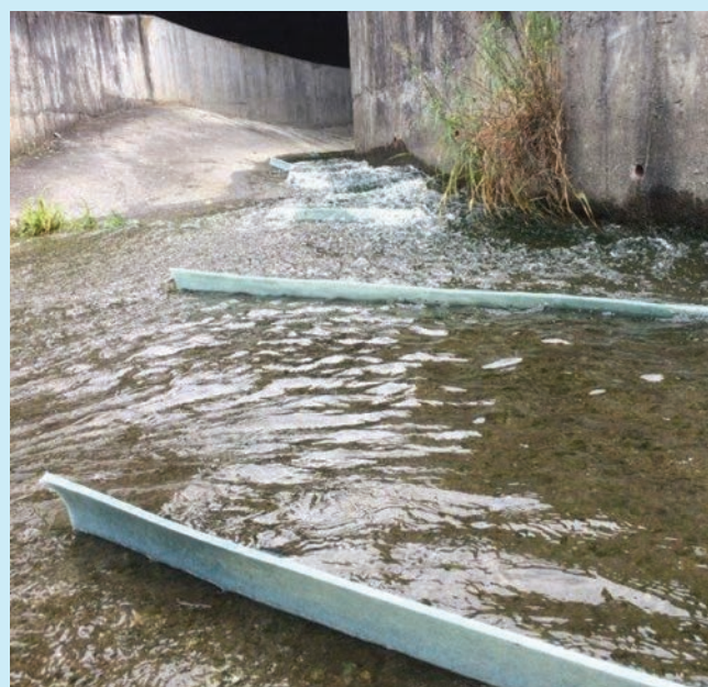
Nile Street underpass. Baffles allow resting pools and slow down water velocity to allow fish to move upstream.
