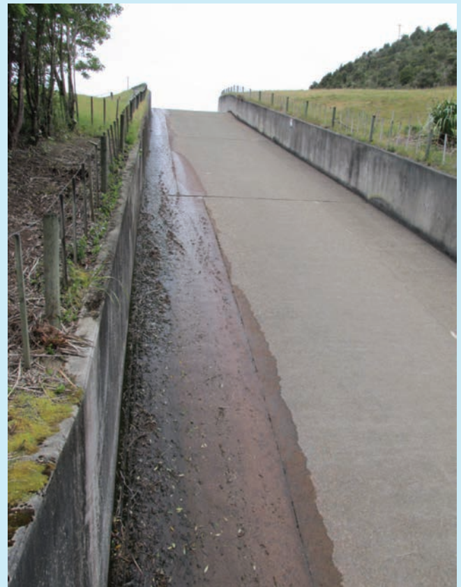
Spat rope and attractant flow at the Maitai Dam spillway.
