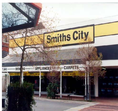
Poorly placed and over-stated signage creates visual clutter...
