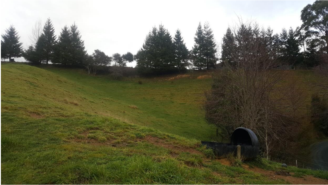
Photograph 5: Looking north east, soil creep at the top of the slope.
