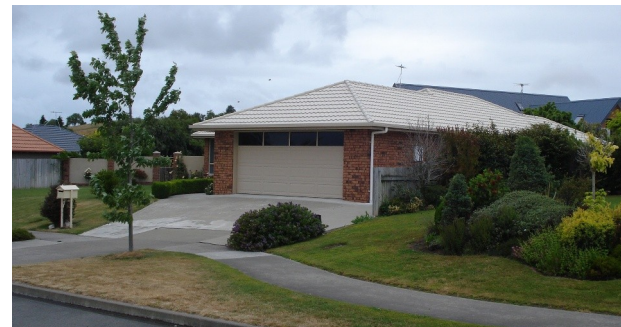
FIG 3: This triple garage set forward from the rest of the house, combined with a large paved area for parked cars, shows poor streetscape.
