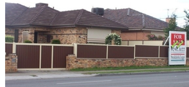
FIG 6: Example of how a high, non-permeable fence, combined with blinded windows results in a poor interface
